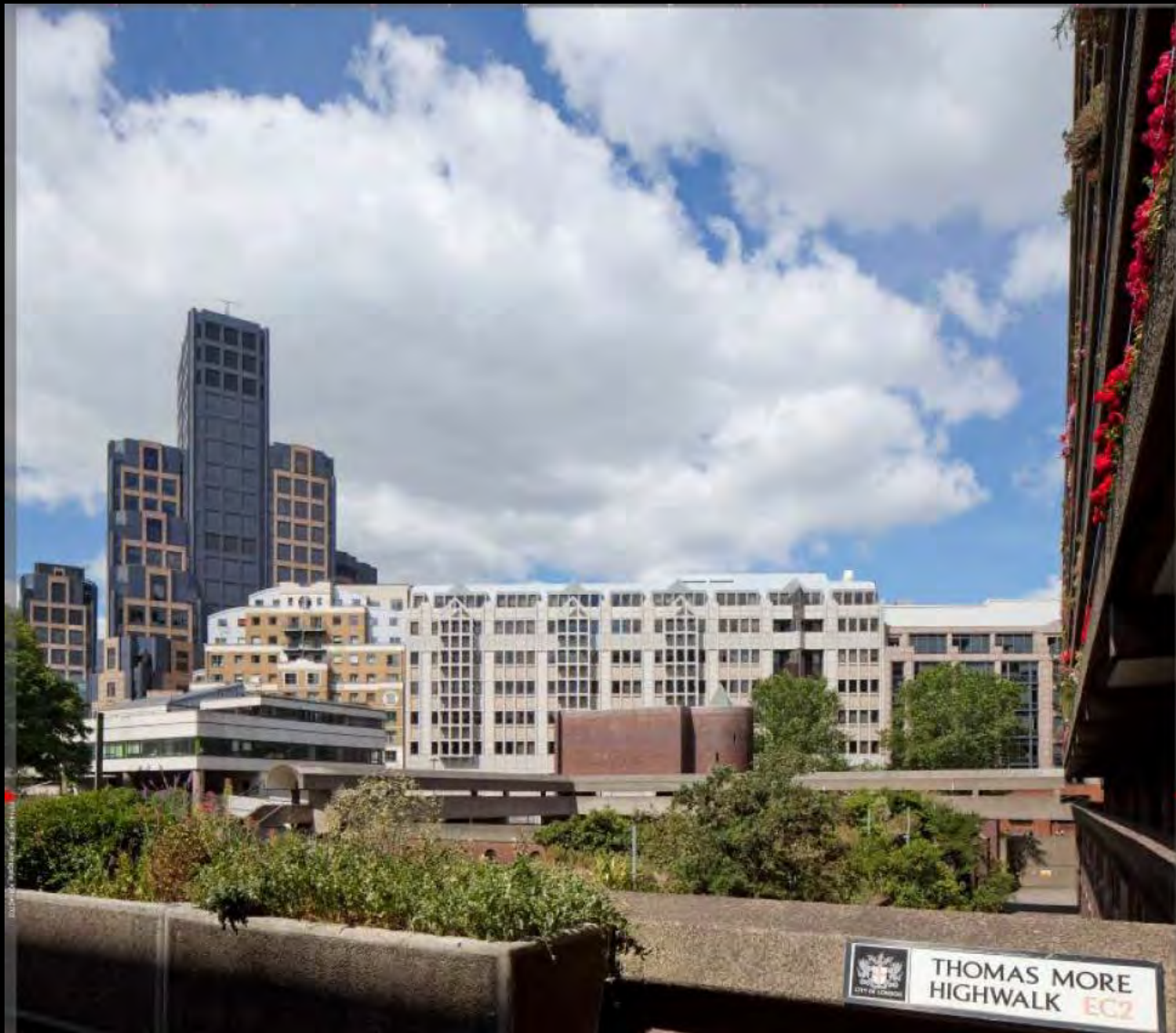
Existing view – from Barbican Estate
