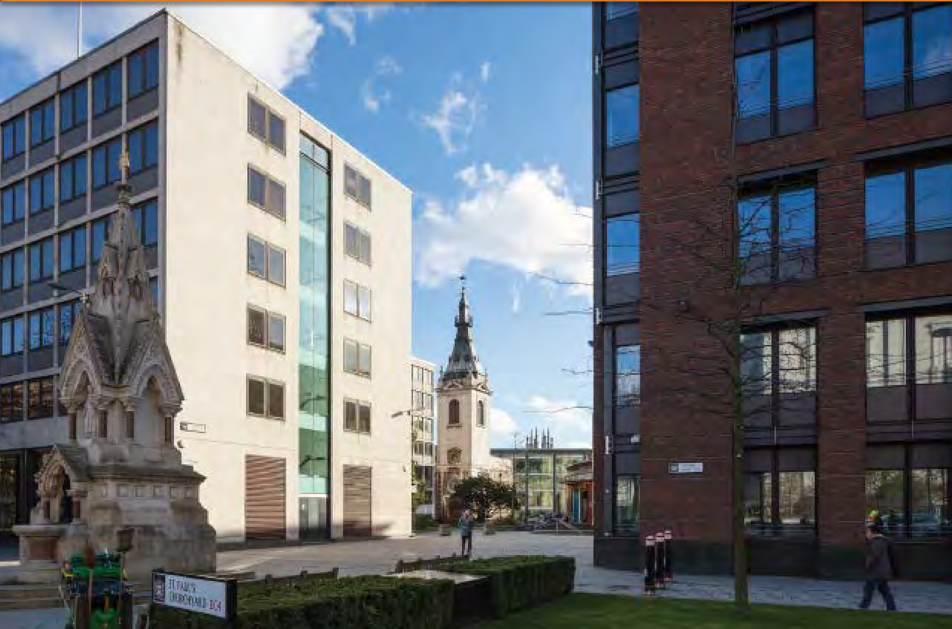
Existing view from southern pavement of St. Paul's Churchyard Gardens
