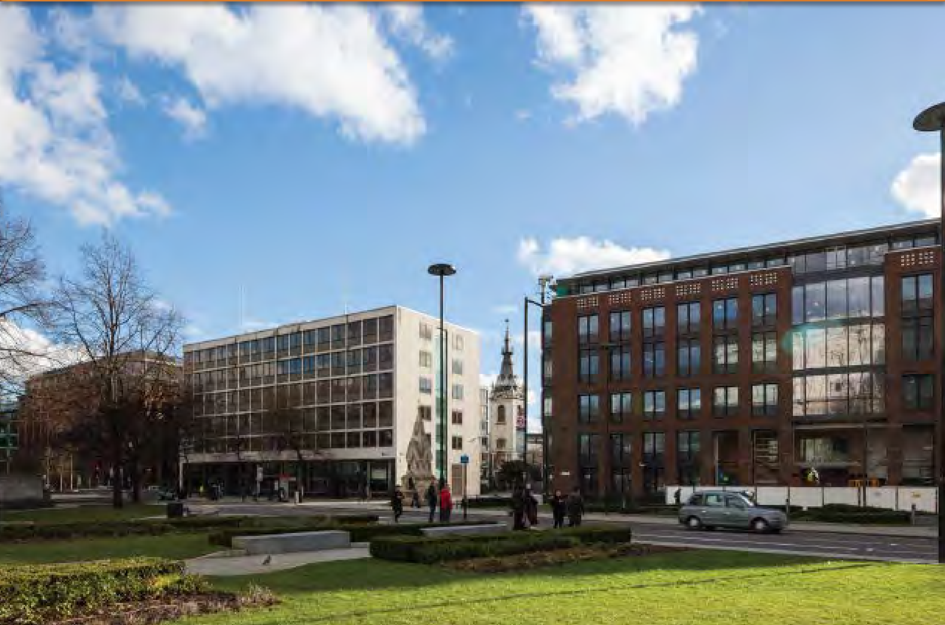
Existing view from St. Paul's Churchyard Gardens
